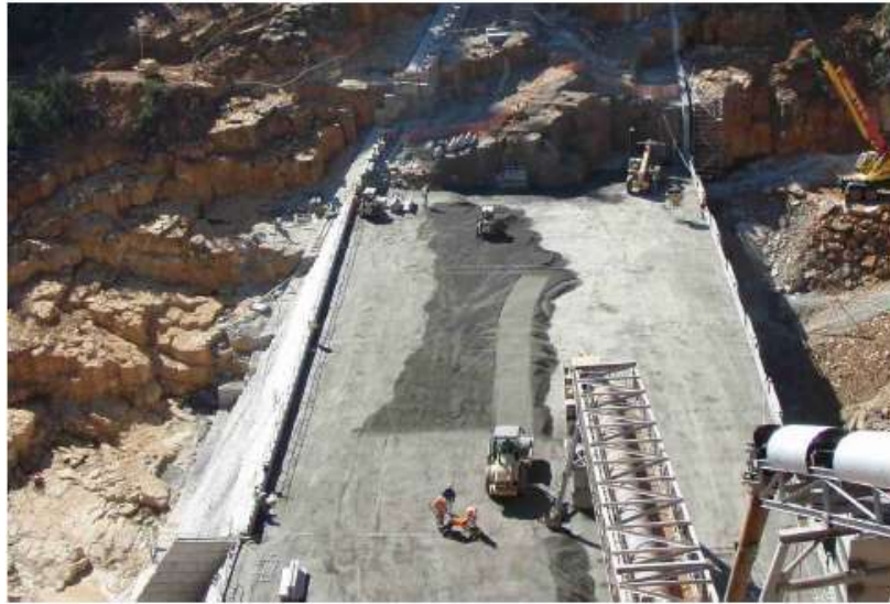
Figure E-0-5 – Example of RCC Dam Construction
