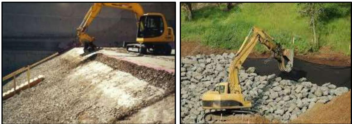
**<Figure 1-19> RCC Dam Slope Forming & Riprap**
