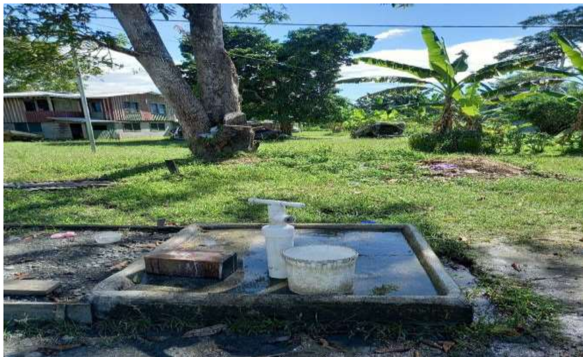
Borehole with hand pump used for community drinking, washing, shower
