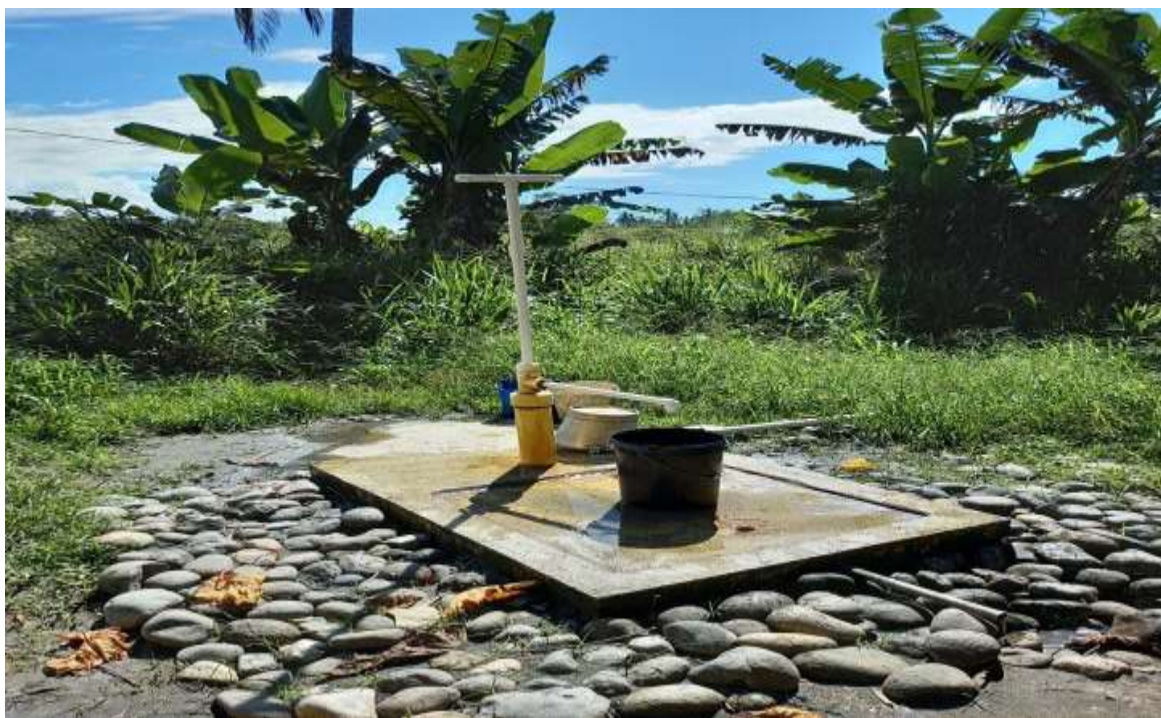
Borehole with hand pump used for shower and washing but unfit for drinking and cooking
