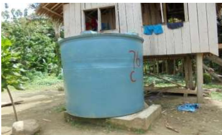
Figure 12-5 Rainwater tank at Pachuki
