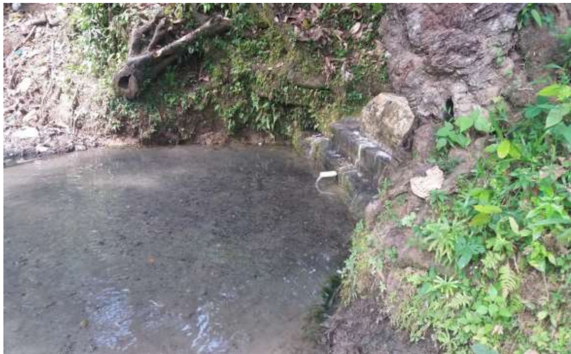
Spring protected with concrete box at Verakabikabi
