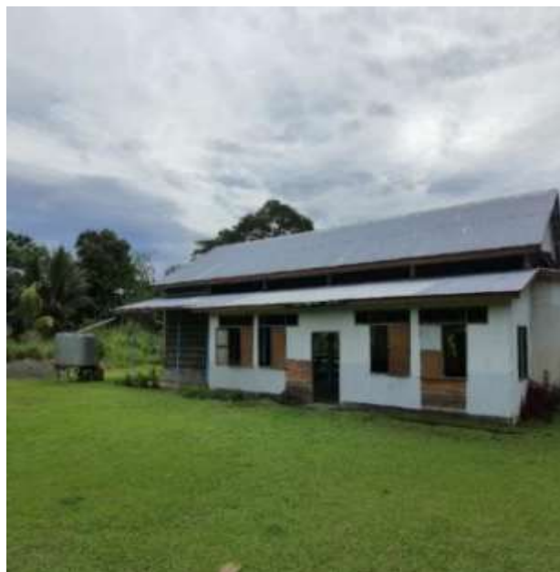
Figure ES-8 Rainwater catchment from church roof, Old Selwyn
