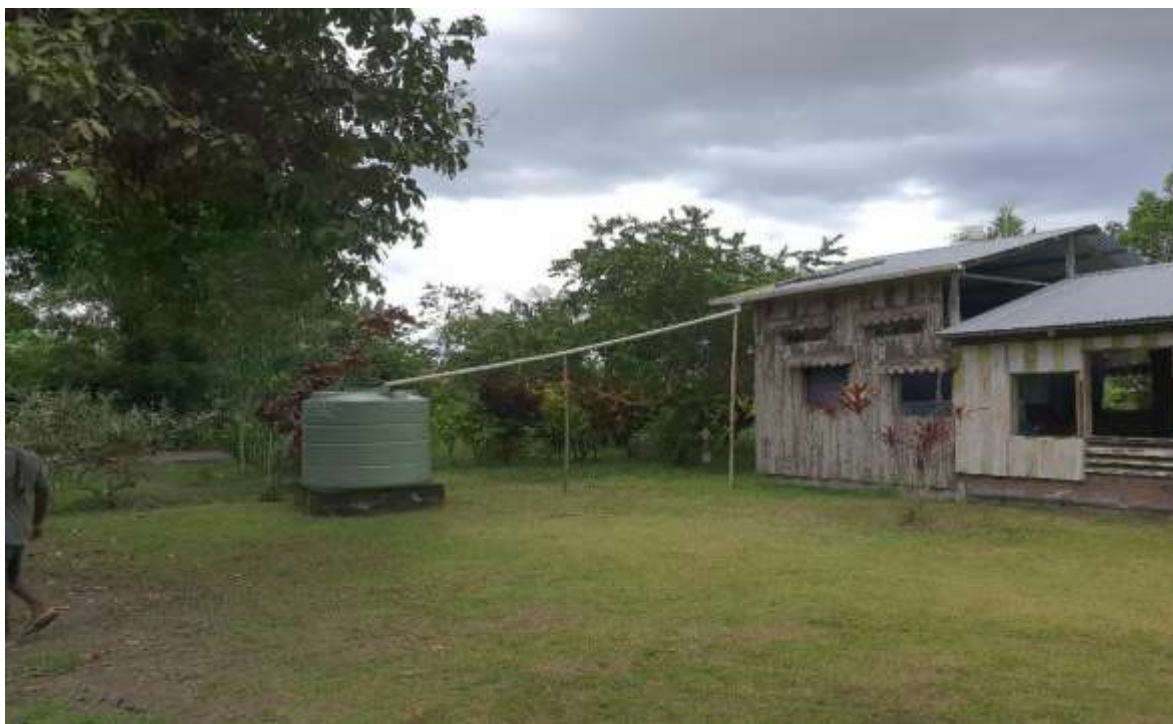
Community Rain water tank installed near the church Building
