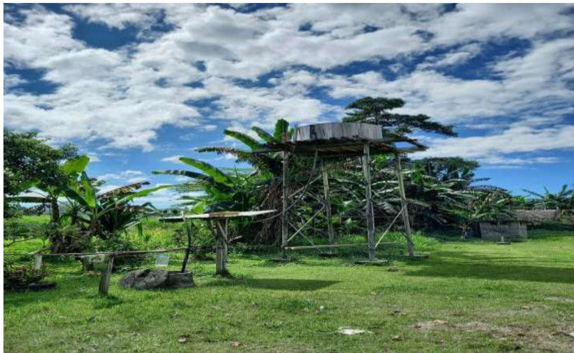
Overhead water storage tank fed from dug well
