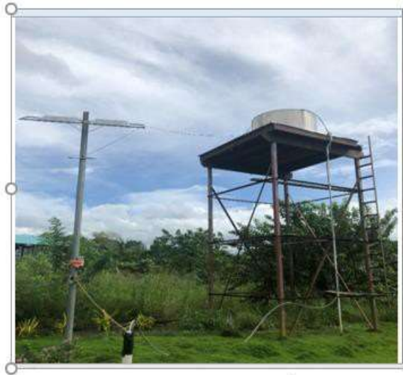
Figure ES-7 Solar pump on borehole at Vera'ande.
