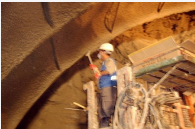
Secondary Shotcrete Placement/
