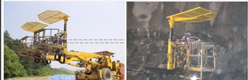
Installing Boards on Top of Bucket
