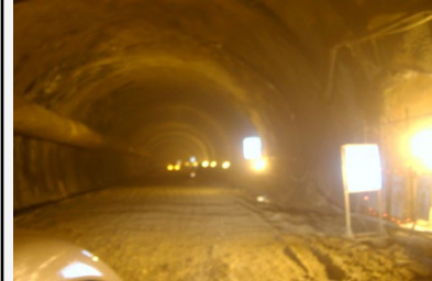
Installing Reflective Safety Signs
