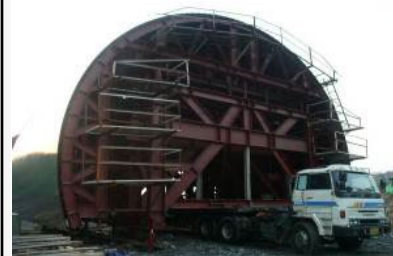
Temporary Safety Facility for Lining Form Fabrication
