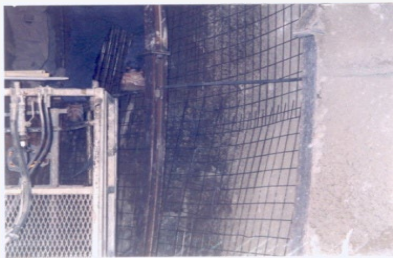
Installing Wire Mesh and Steel Ribs
