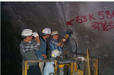
Rock Bolt Construction
