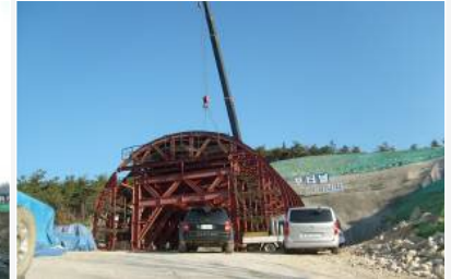
Temporary Safety Facility for Lining Form Fabrication
